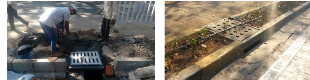
Horizontal opening along the saucer drain
