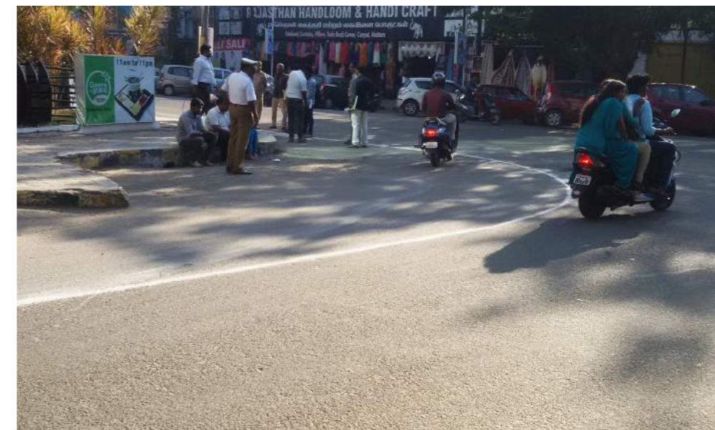
Fig. (above) Kerb line marking in a street in Chennai
