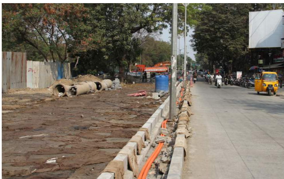
Fig. (above) Tilling of carriageway in FC Road, Pune
