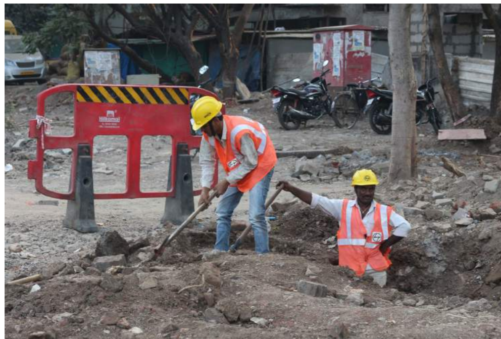
Fig. Street edge under construction on ITI Road, Pune
