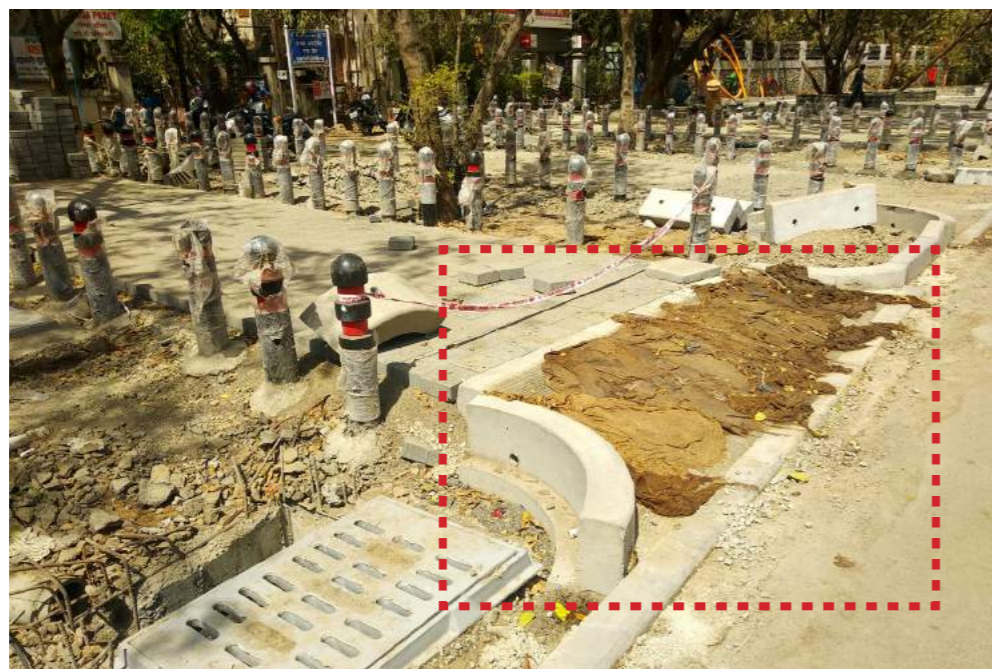
Fig. (top) Property ramp with flaring on both sides
