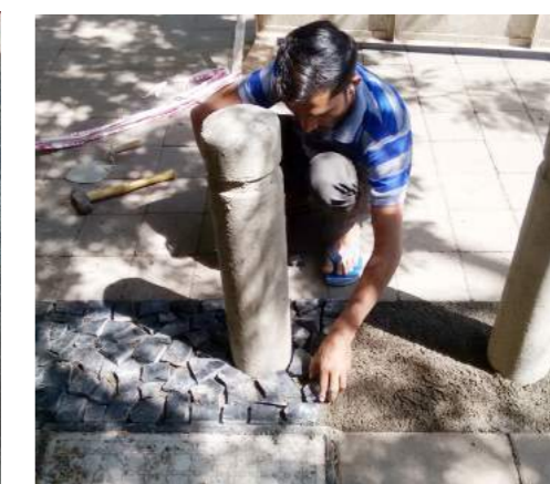
Fig. (top) Fixing of bus shelter in Pune
