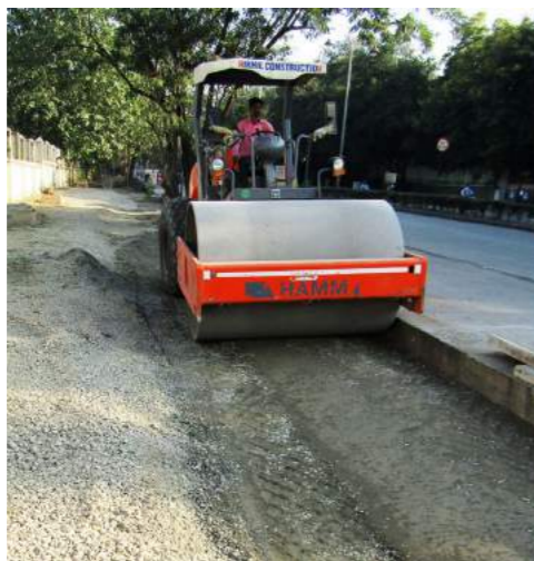
Fig. (top) Utility bed preparation and backfilling in FC Road, Pune
