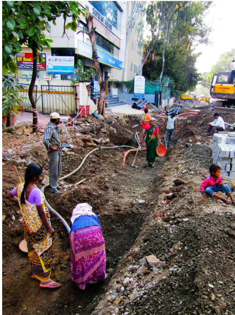
Fig. Subsurface work in progress in FC Road, Pune
